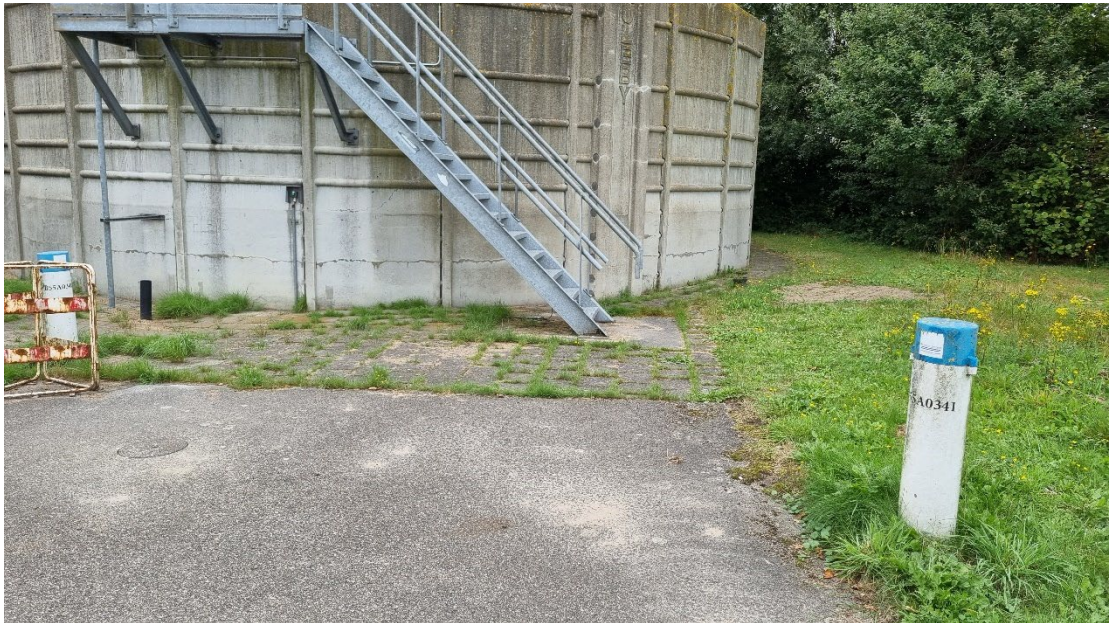
Figure 3.5: Wells B55A0340 and B55A341 at the wastewater treatment plant of Hulst. The photo is taken towards the east. The numbering on the wells indicate that B55A0340 is in the north, while B55A0341 is in the south. However, the map of Vermoortel et al. (1996) indicates that it should be the other way around.
