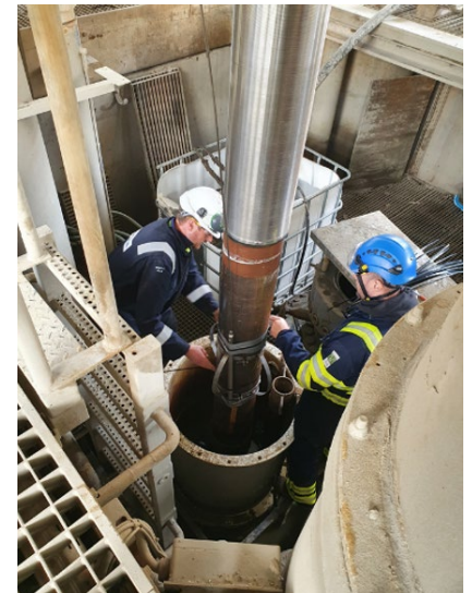
Figure 20: Full operational drill rig with 2 research wells 450 meters deep at Rijswijk Centre for Sustainable Geo-energy
