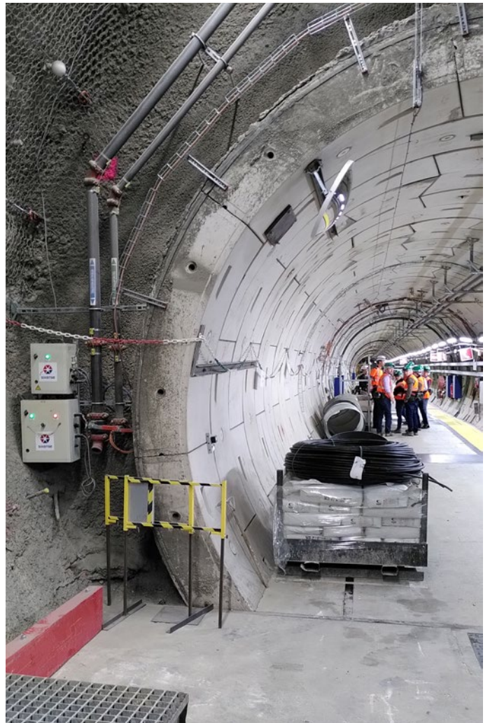
Figure 2-5: Constructed parts of underground facilities with segmented concrete liners in poorly indurated clay (left; source EURDICE) at 225 m depth in Mol (Belgium) and in indurated clay (right) at 490 meters depth in Bure (France).
