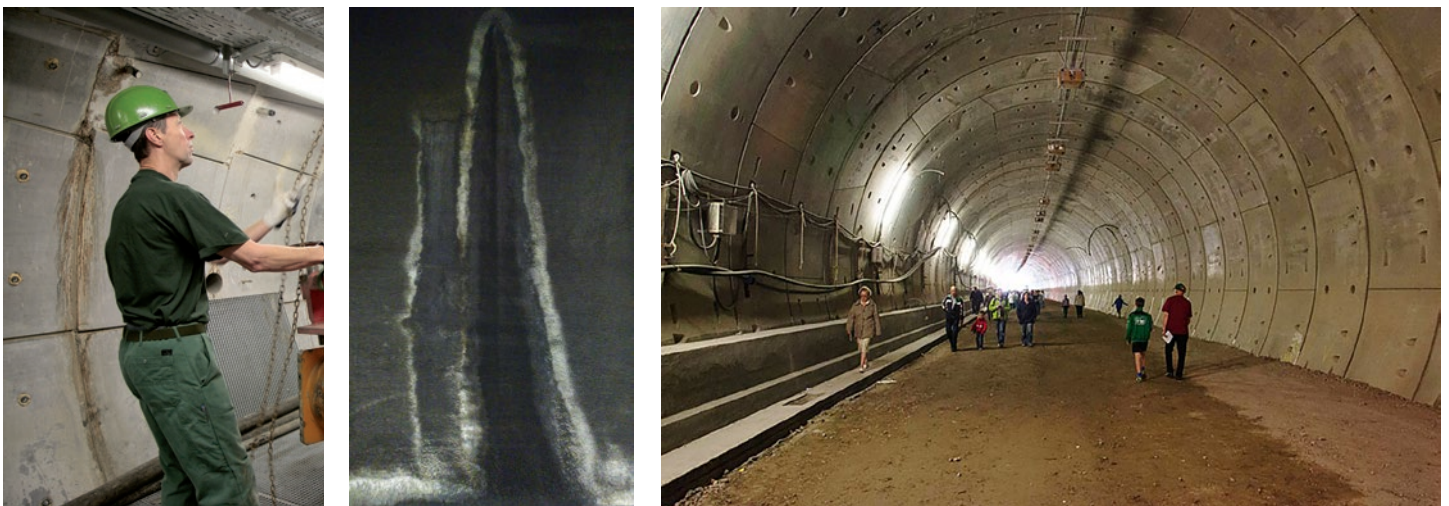
Figure 4-9: Salt deposits at joints of concrete segments in the Belgian URF (left) and Dutch traffic tunnels - Westerschelde (middle) with whitish deposits and Sluiskil (right) with joints between segments in the top, no salt deposits yet. All tunnels have been constructed in Boom (Rupel) Clay.
