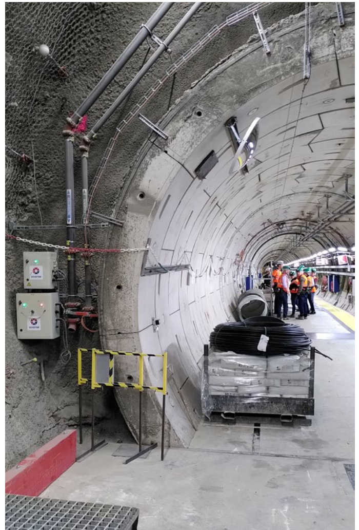
Figure 2-5: Constructed parts of underground facilities with segmented concrete liners in poorly indurated clay (left; source EURDICE) at 225 m depth in Mol (Belgium) and in indurated clay (right) at 490 meters depth in Bure (France).
