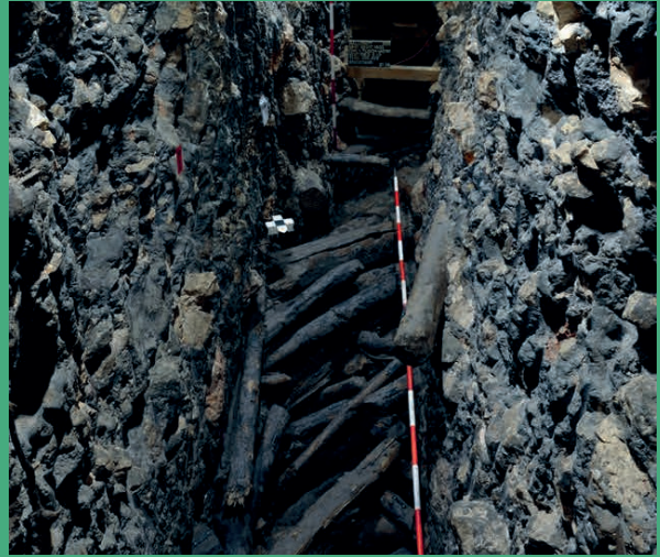
Figure 1) Fractured mine timber in the Hallstatt salt mine. This wood is over 2,000 years old and is exceptionally well preserved. Photo taken by D. Brandner, NHM Vienna and is from Reschreiter and Kowarik (2019).
